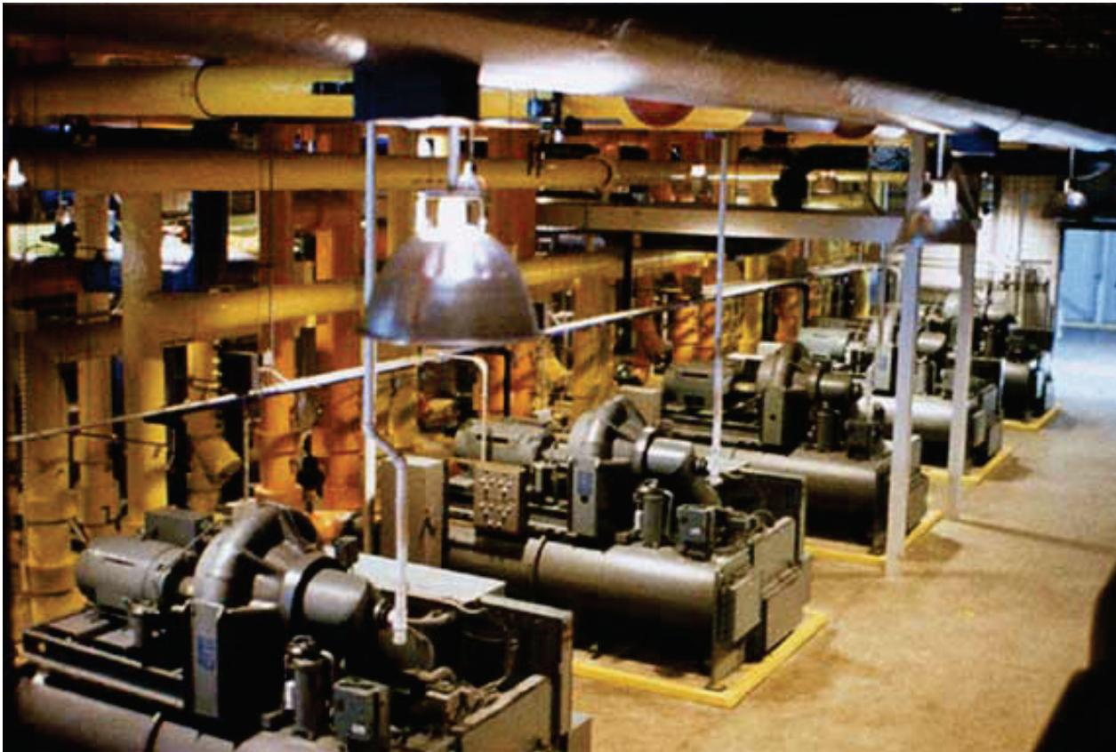
These pumps are used to pump the heated water to buildings in a district heating system, after it has passed through the heat exchanger.
