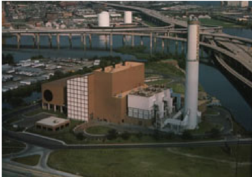
Baltimore RESCO (Refuse Energy Systems Company) Plant Russell Street & U.S Interstate 95 (shadow of Ravens Stadium)
