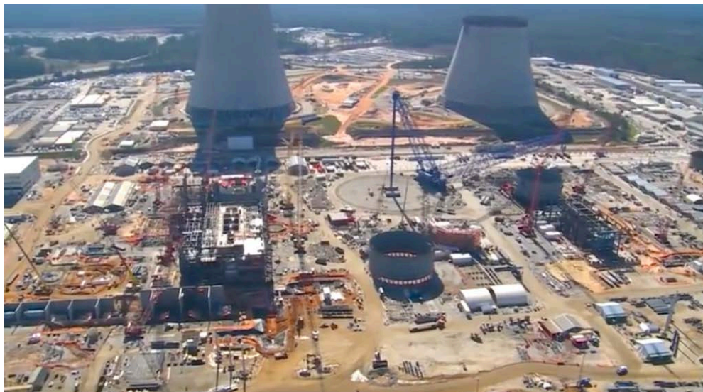
Vogtle 3 & 4 under construction. Source: Southern Company
