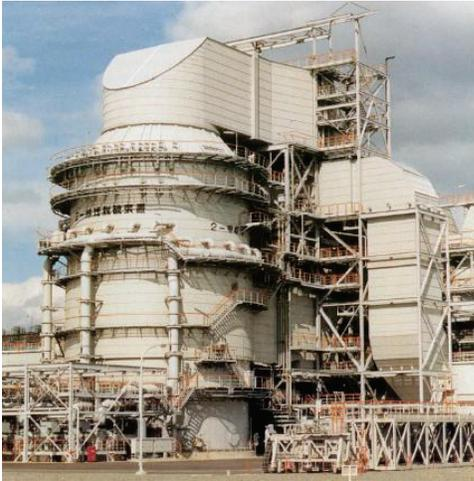
Pulverized limestone (CaCO<sub>3</sub>) is mixed with water to make a slurry sprayed into flue gas, resulting in:
